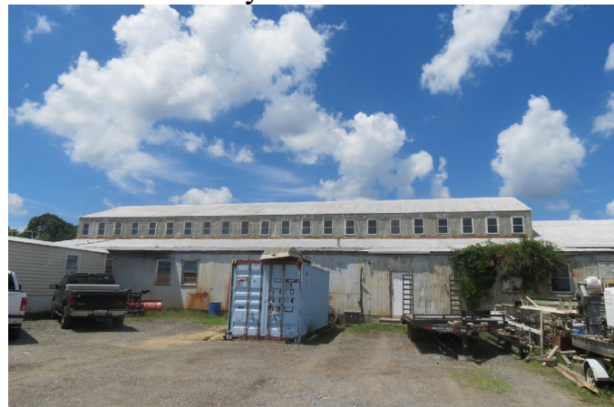
Washburn’s Boat Yard Shop Building Inside Washburn’s Shop Building. Note the Lifting Trolley I Beam tracks.
