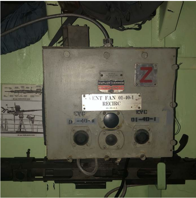
The fan control box in process of being connected in the original location in the Clipping Room beneath fan.
