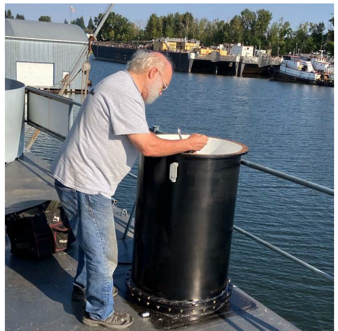
Installing wiring conduit up through the deck.
